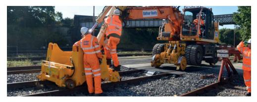
ur E-Clip De-Clipper is the ideal solution for the rapid removal of Pandrol E and PR clips.
